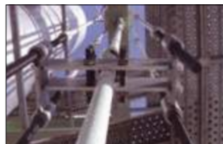
Installation of load evaluation devices
