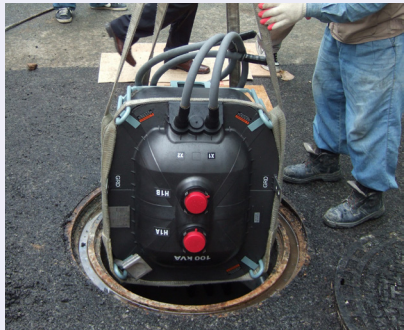
KEPCO / Korea Installation in a manhole
