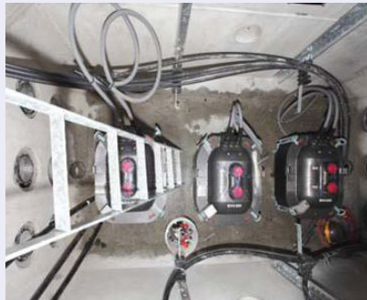
KEPCO / Korea 3PH installation in a manhole
